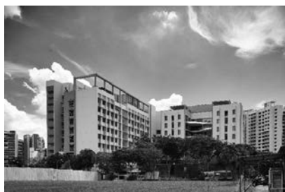
Nursing Home at the North of Singapore
